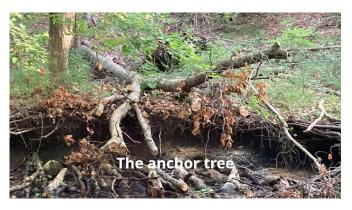
Next the hoist went to work on a large boulder (~3-4 foot diameter) which was dragged from the middle of the river and up against the tree to lock it into place. Next a couple of smaller boulders were similarly dragged into place firmly anchoring the tree to the bank. Jeff then gave us directions on how to perform the next step to backfill the other side of the tree with cobble dug up from the stream channel. He showed us how
